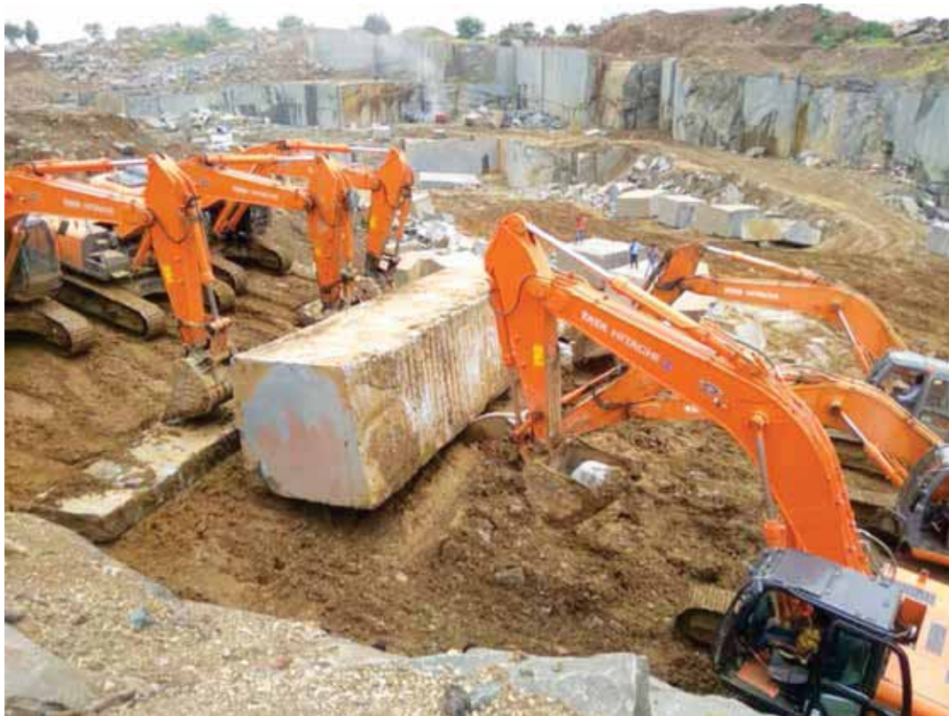
Stone being moved with excavators at the quarry in Chirumadaram, district Khammam, Telangana.
