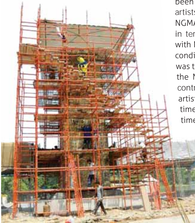
Scaffolding around the stone for NGMA artists to work.
